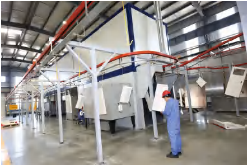
Automatic powder coating lines
