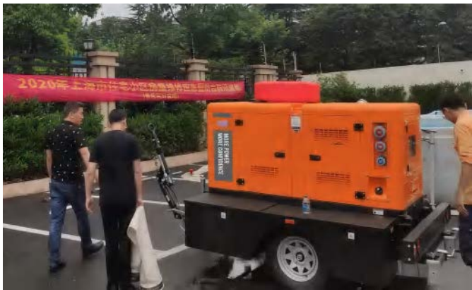
Shanghai, Perkins, Emergency
