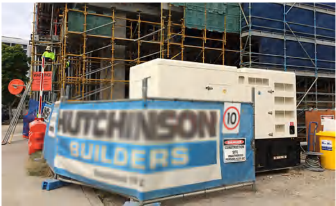
Puerto Rico, Cummins, Construction
